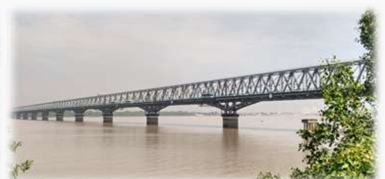
➤ Thanlyin Bridge (Myanmar)
