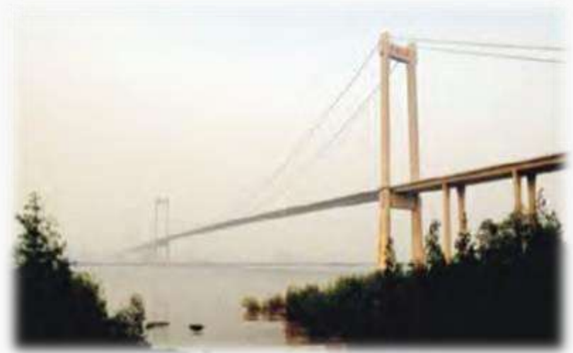
➤ GuangZhou Pearl River HuangPu Bridge
