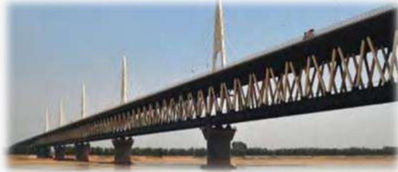
➤ ZhengZhou Yellow River Bridge
