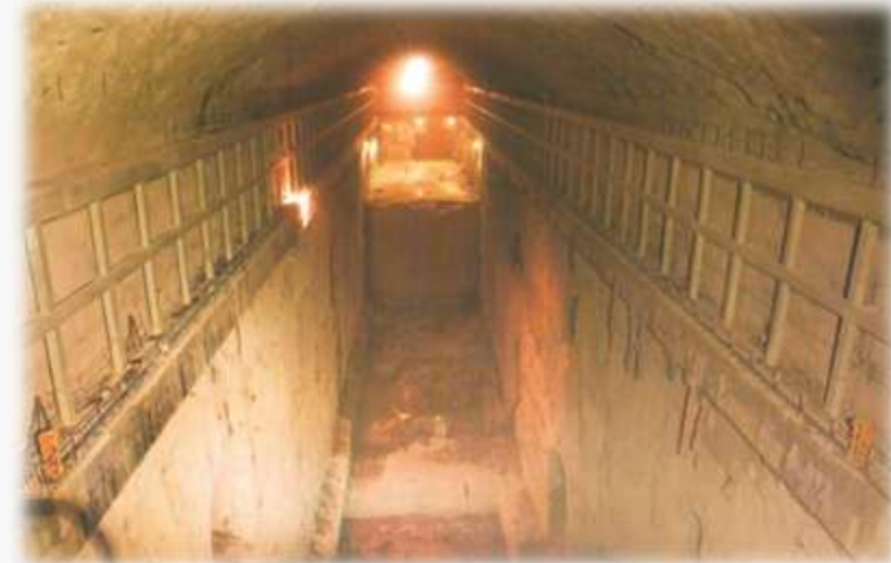
•Huangdeng Hydropower/ Yunnan
