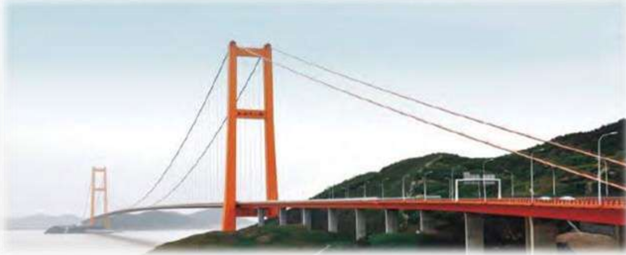
➤ ZhouShan XiHouMen Bridge
