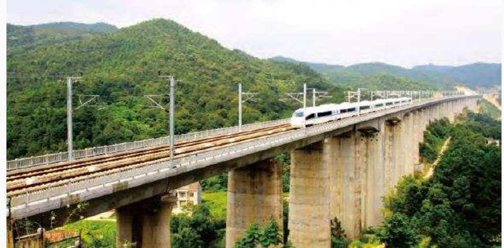
•Shanghai – Kunming High Speed Railway
