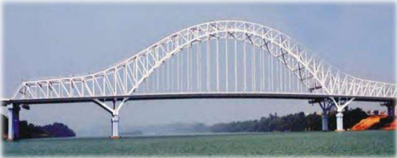
➤ GuangXi LouZhou WeiYi Bridge
