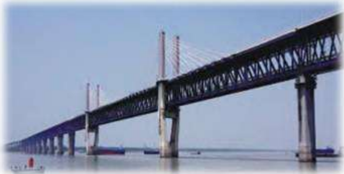
➤ WuHu Yangtze River Bridge
