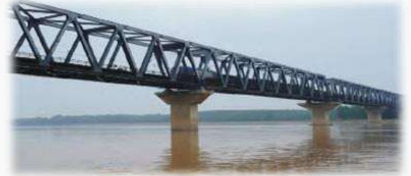
➤ SunKou Yellow River Bridge
