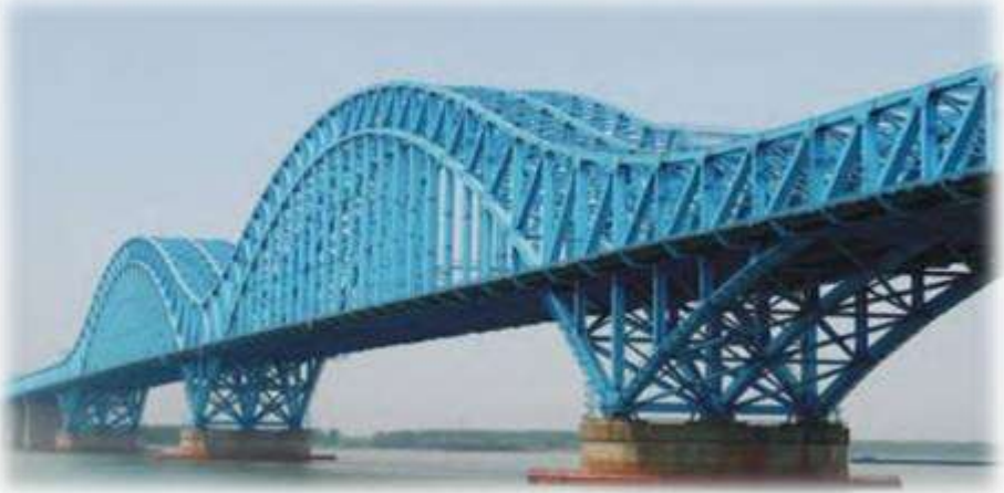
➤ NanJing DaShengGuan Yangtze River Bridge
