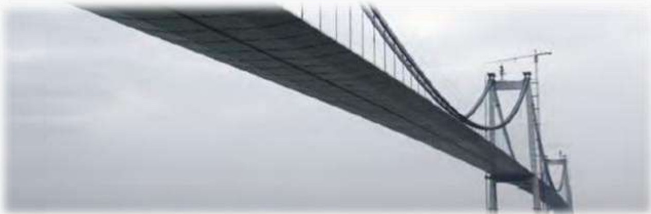
➤ TaiZhou Yangtze River High-Way Bridge
