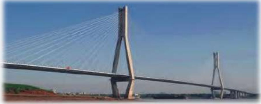
➤ AnQing Yangtze River High-Way Bridge
