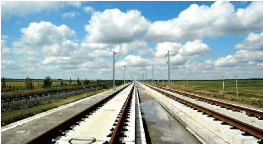
•Ballast-less truck slab High Speed Railway Line
