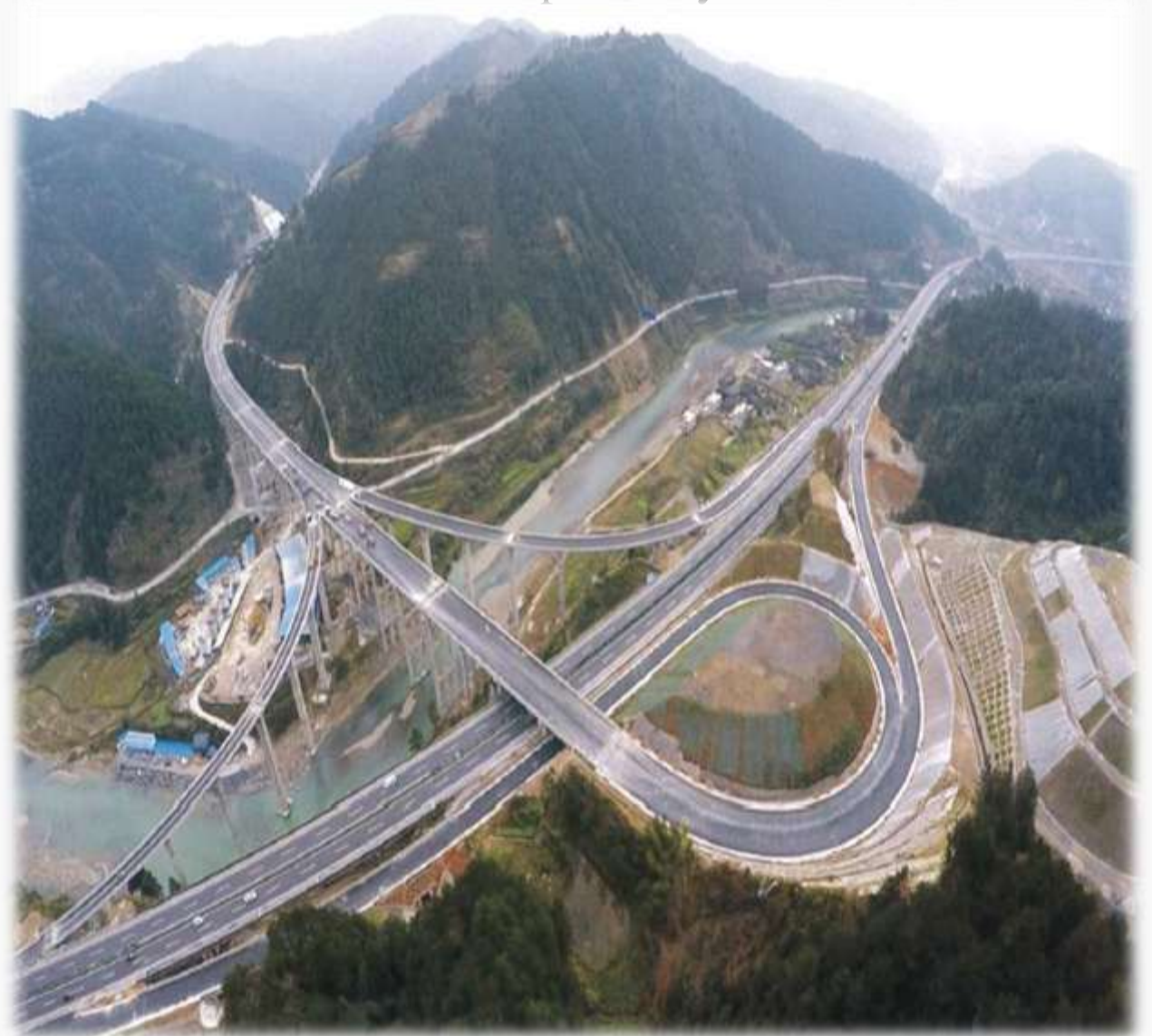
•Kaili – Leishan Expressway / Guizhou
