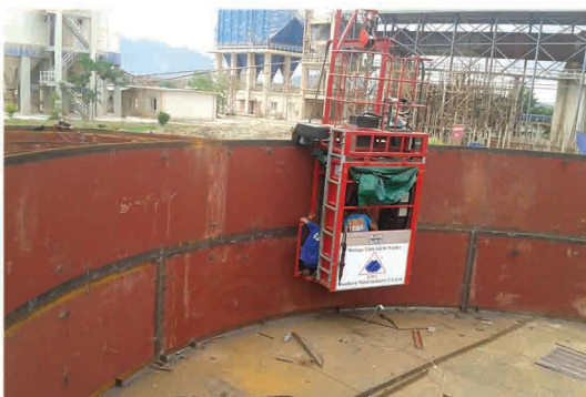
Storage Tank Welding Machine
